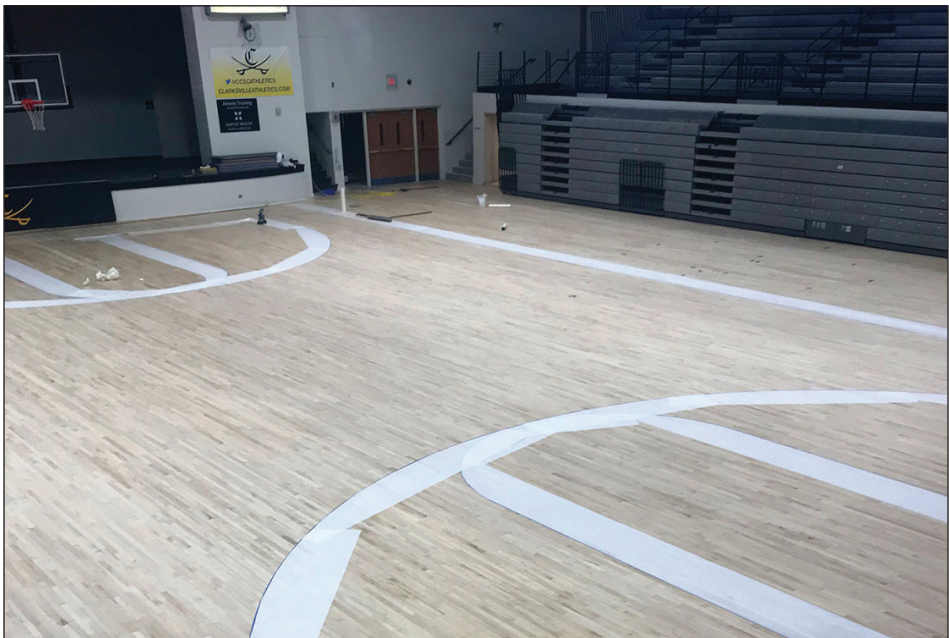
The floor after being sanded down to the bare wood. photo by CHS Athletics
